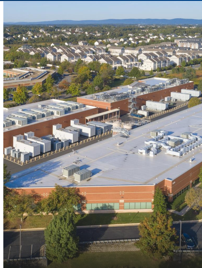
Chantilly Data Center Washington, D.C.
